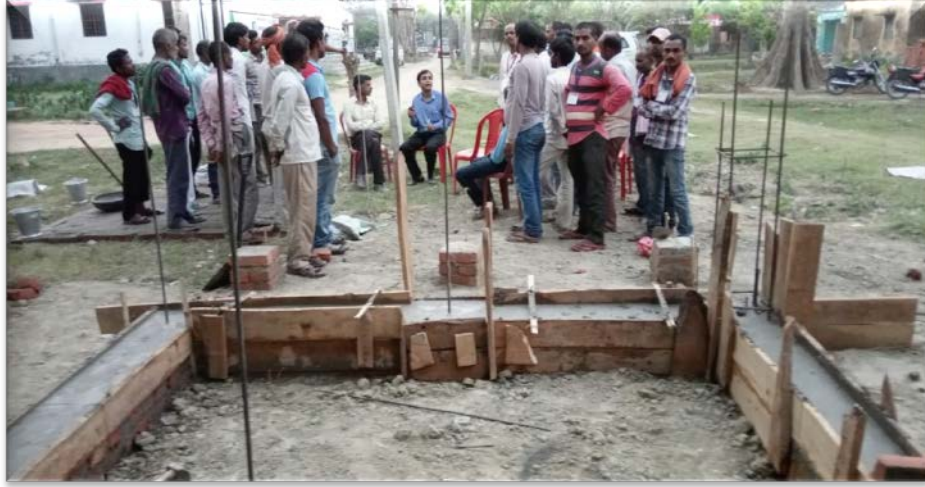
Mason Training on 02 to 08 April 2019 at Sitamarhi District
